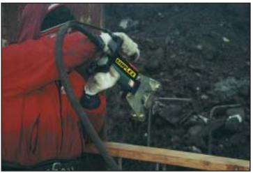
At home on any construction site, the Pow'r-Buddy™ starts and runs reliably on long extension cords. This rebar bending application is no challenge for the Simplex industrial grade pump design. "Easy to carry and simple to use, the Pow'r-Buddy™ helps us through tough construction jobs without problems."
