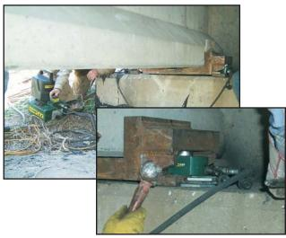
Simplex RFS Series are designed specifically for near impossible lifting, clamping or positioning jobs where space is at a premium. Ideal for break loose or start up spreading jobs. These mini-monsters pack up to 150 tons of force into a convenient, portable package.
